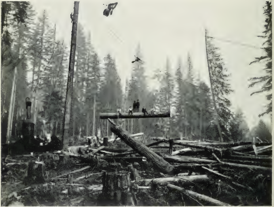
FIG. 56. HIGH LEAD OVERHEAD SKIDDING. [By courtesy of British Columbia Government.]
